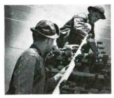
Care must be taken not to damage insulators while stacking crossarms.
