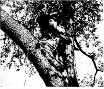
After cable is put fast in position and circuits are ready for test, these men go into action. Note portable phone set.
