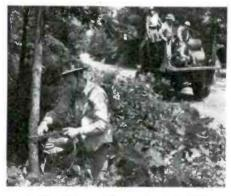
A Signal Corps lineman tying field wire in place prior to stringing.
