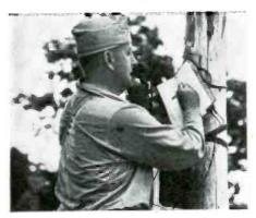
Outpost field telephone straps around pole or other supports.
