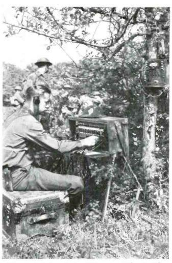
Closeup view of twelve-line field type switchboard. The instrument mounted on the tree is wire chief's testing set.
