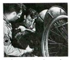
Servicing a wire reel cart used in stringing communication lines.
