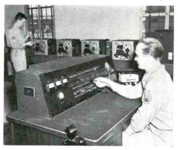
Code from the many tape machines are fed to this control panel where signals are fed to various classrooms.
